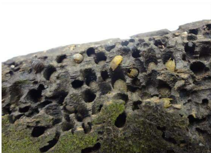
Attack of Sphaeroma terebrans on the wooden piles of Kg Ayer in the Sg Brunei
